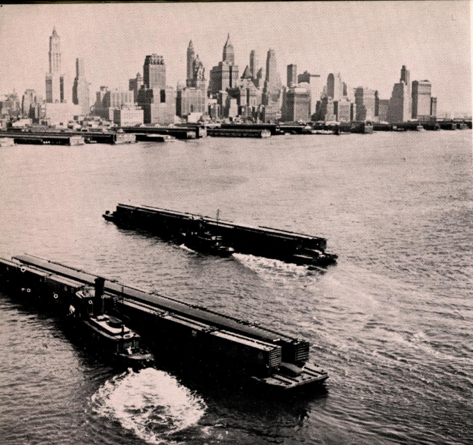
With a background of the awe-inspiring New York skyline, rail cars loaded with fresh fruits and vegetables are floated from Jersey City terminals across the Hudson River to the Manhattan pier location of the New York Fruit Auction Corporation.
